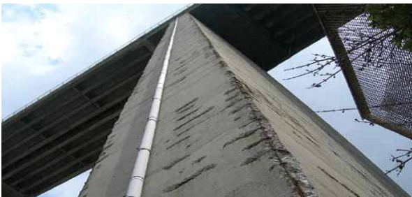
Fig.2. Aggression by CO 2 of an industrial building
