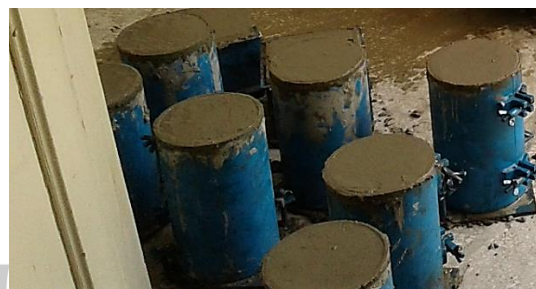
Figure 1: Casting of Concrete
