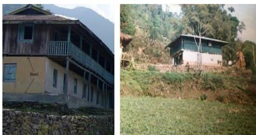
Figure 17: Composite timber first floor supported by brick masonry(left) and rammed earth (right) in ground floor
