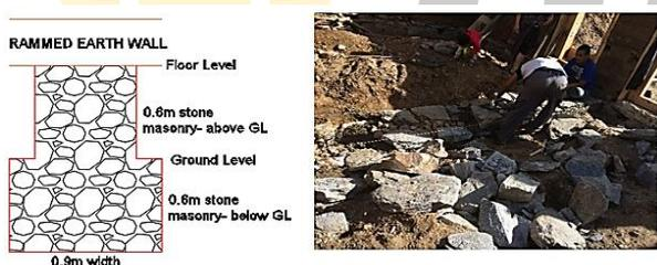
Figure 3: Foundation section (left) and work execution (right) for rammed earth houses.
