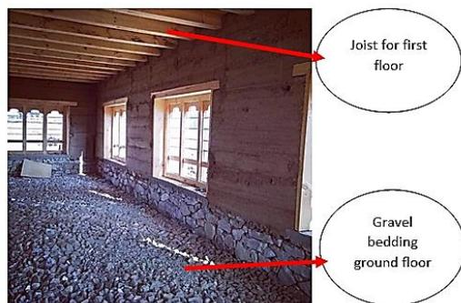
Figure 5: Gravel bedding for first floor and joist for second floor visible
