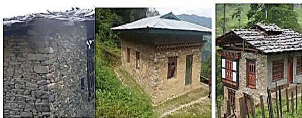
Figure 8: Various Type of stone masonry structure in eastern Bhutan (MOWHS)
