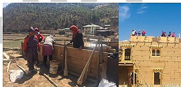
Figure 4: Shuttering for wall erection (left) and rammed earth wall compaction process (right)
