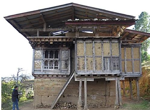
Figure 15: composite wattle and daub over rammed earth ground floor (João M. Guedes et al).
