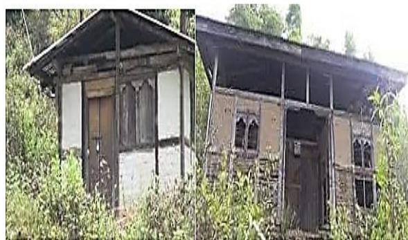
Figure 14: Wattle and daub house (left) and old remains of wattle and daub house (right)
