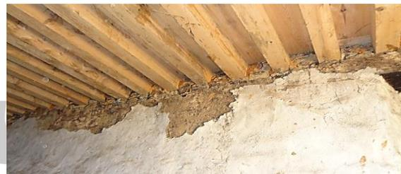
Figure 11: Timber joist over stone masonry wall
